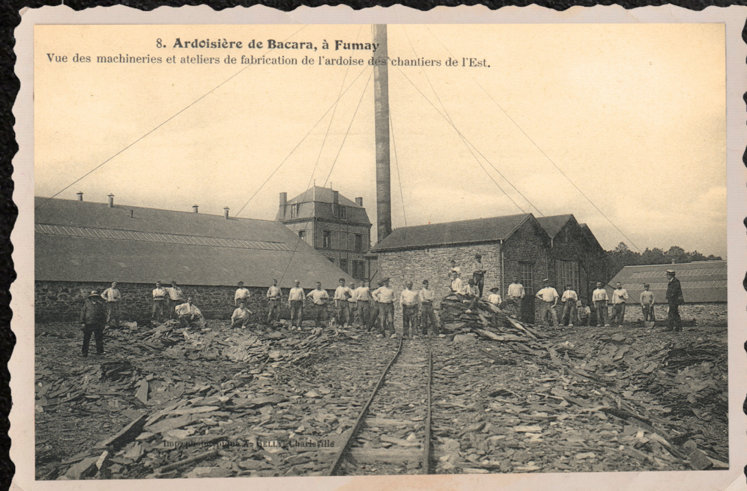
New construction projects at the slate mine
