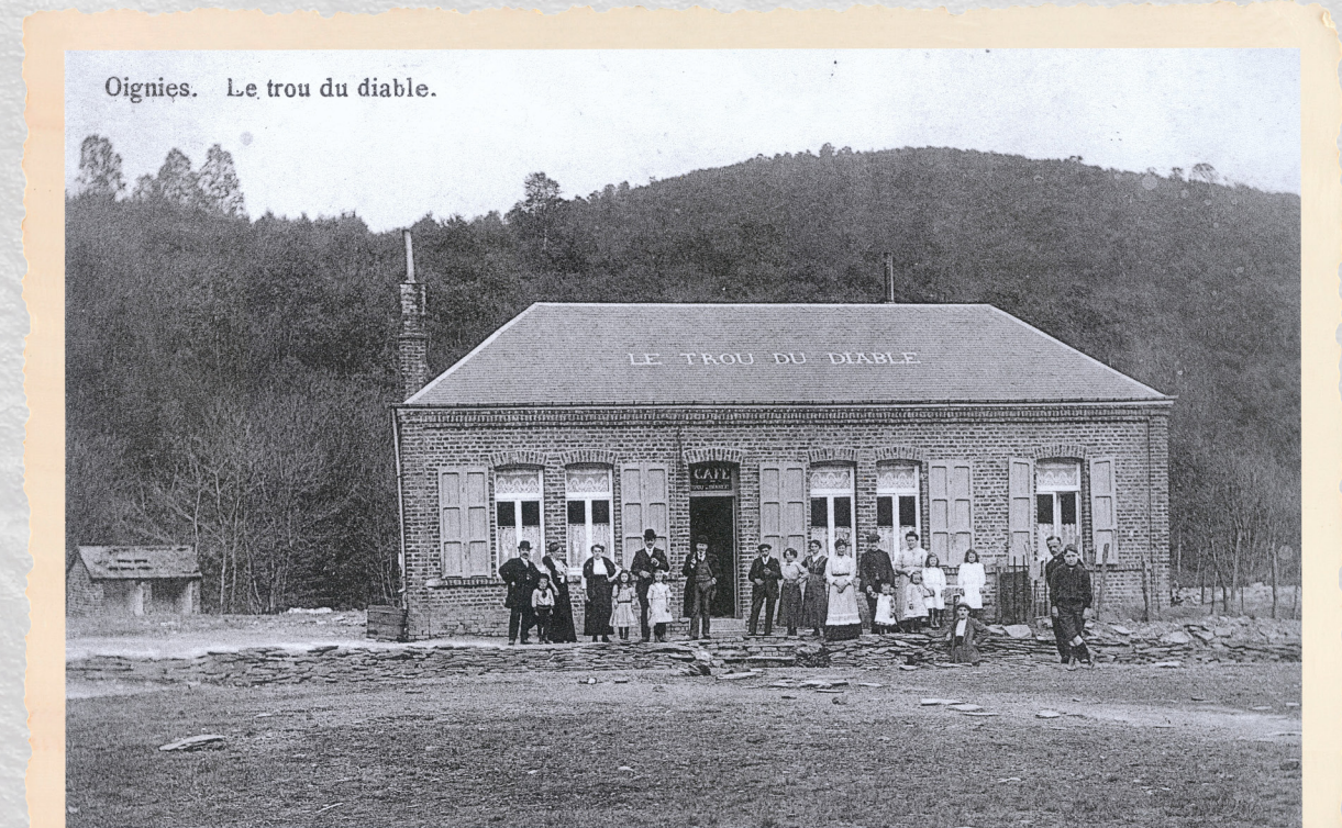
Office and Cafe opposite the Trou du Diable slate mine
