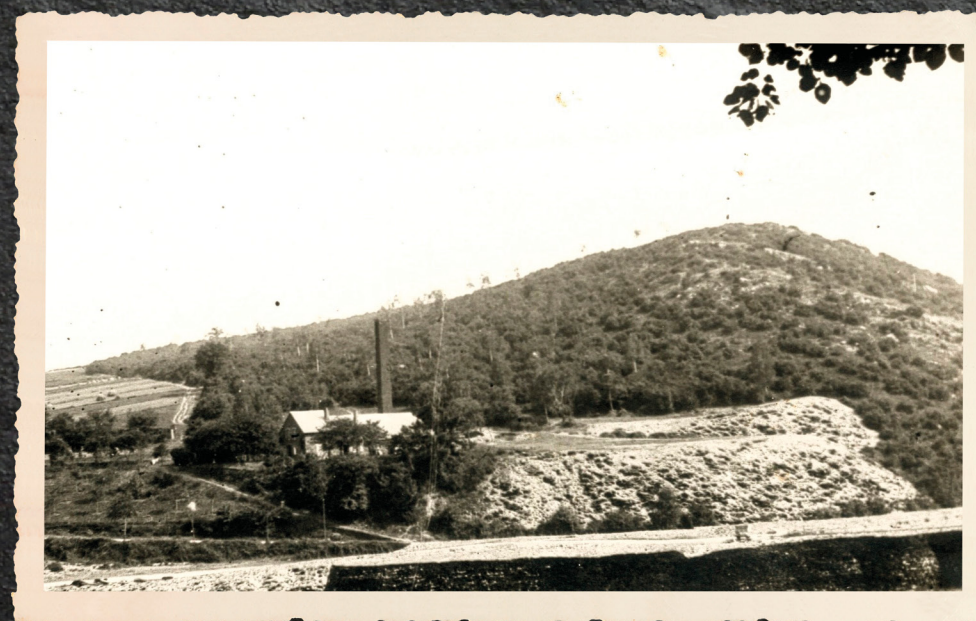
Saint-Lambert slate mine
