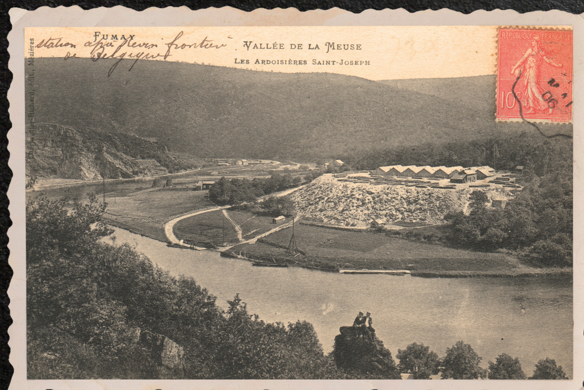
Overview of the slate mine at the beginning of the 20e century
